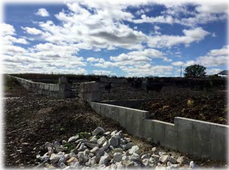
Waste Containment Area
