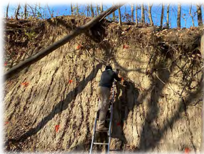
Installation of Bank Pins
