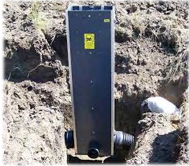
Water Control Structure
