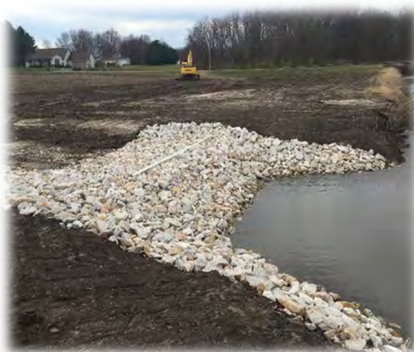
Grade Control Structure – Block Chute
