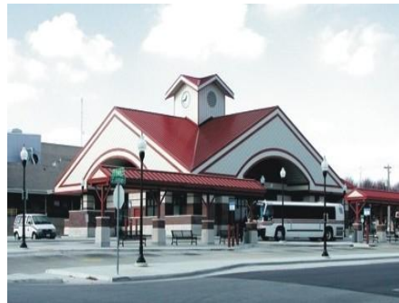
DPTS Senator Severns Transit Center
